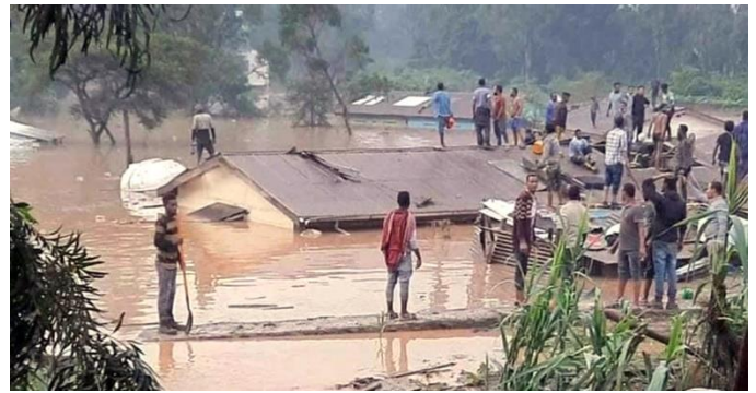
Faculty housing on the campus of the seminary of Ethiopian Evangelical Church Mekane Yesus (EECMY) in Addis Ababa, Ethiopia, is shown submerged in floodwaters following heavy rain and the failure of a dike on Aug. 15, 2021. Rebuilding is underway with assistance from a mercy grant from The Lutheran Church—Missouri Synod. (Photo courtesy of LCMS Africa)
